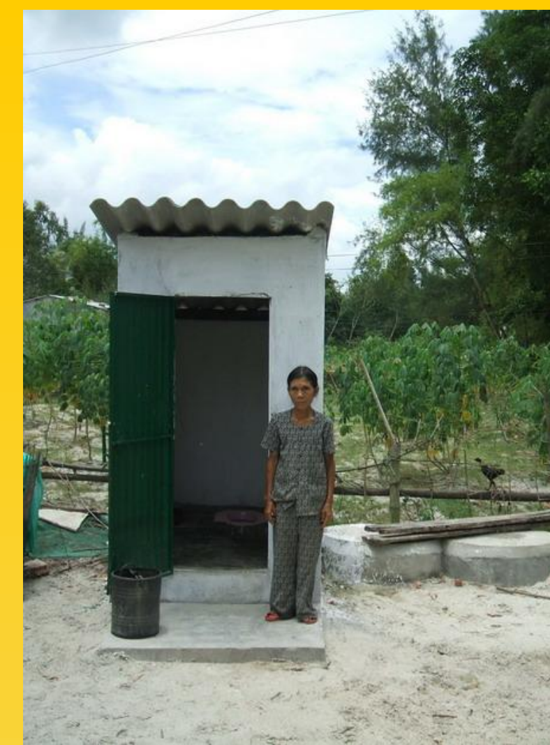
Fig 4. Model of semi-septic pour-flush toilet facility supported by OBA rebate.
