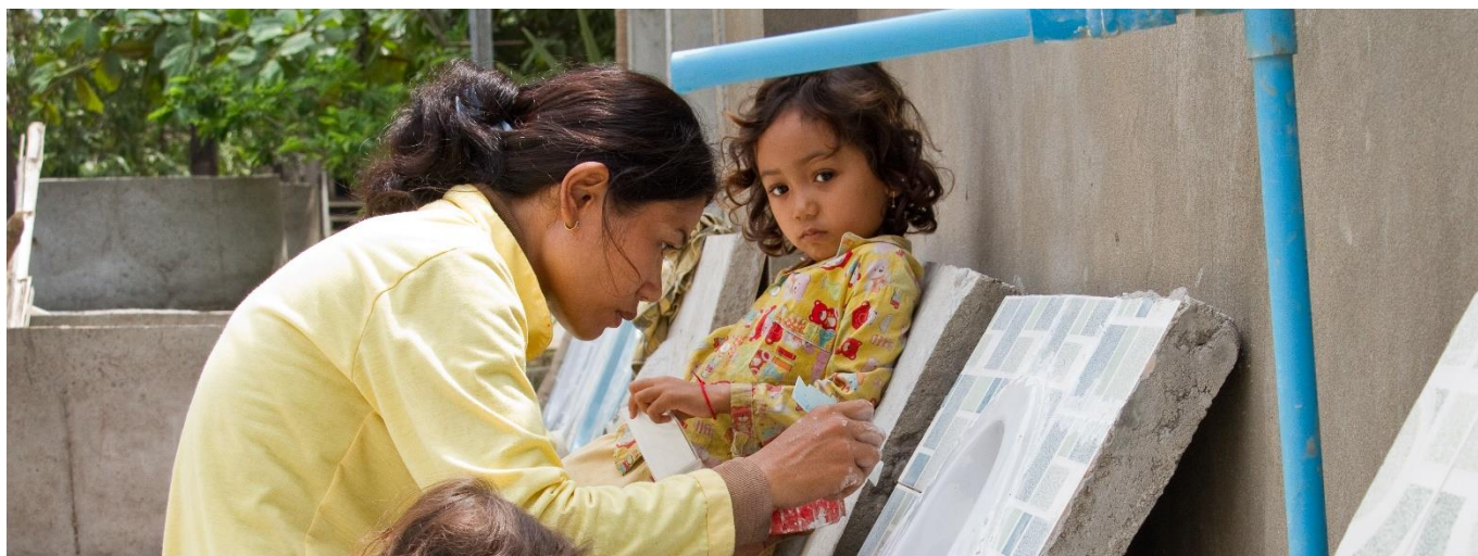
Local supplier tiling a squat toilet slab (Credit: WaterSHED)
