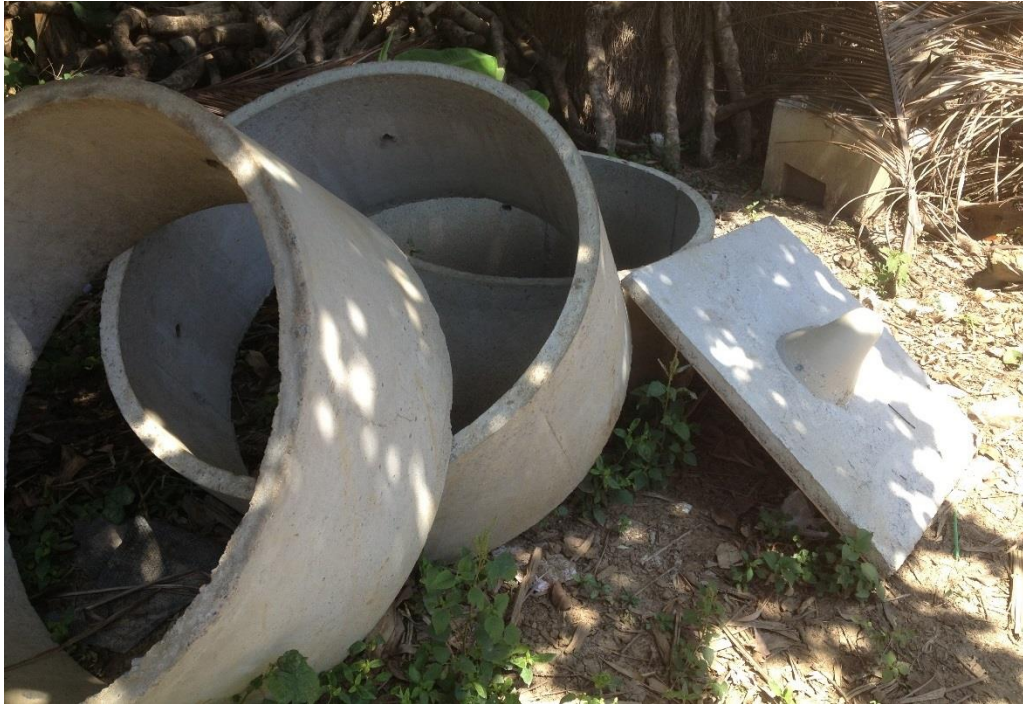
FIGURE 4 CORE LATRINE COMPONENTS AWAITING INSTALLATION
